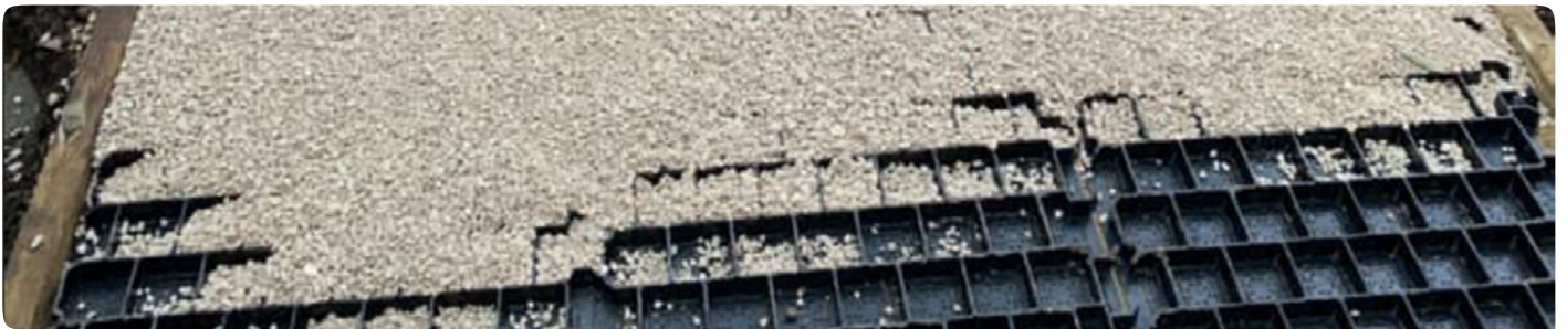
CORE TRP base during installation
