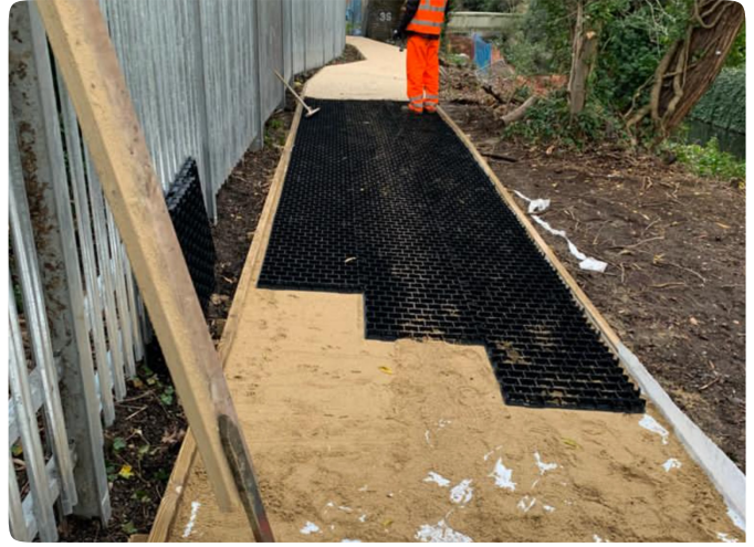
CORE COMMERCIAL Gravel Grid overlay
