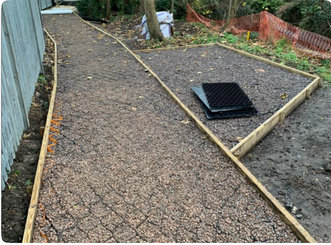
CORE TRP base during installation
