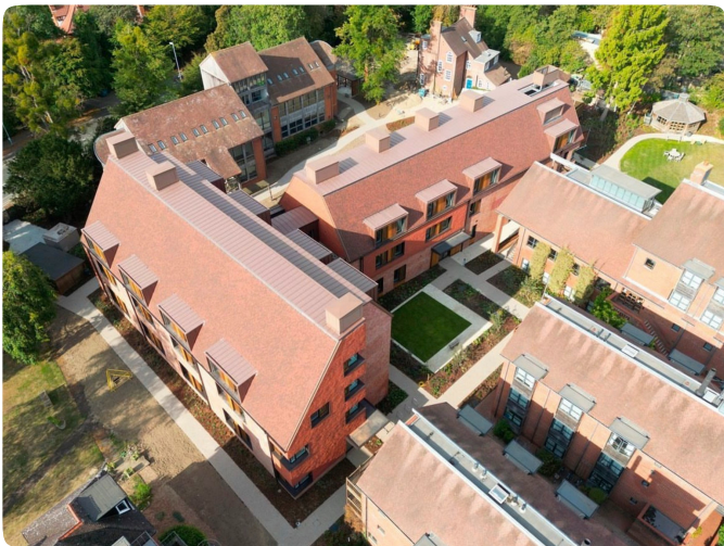
Courtyard paths connect the new building with its setting.
