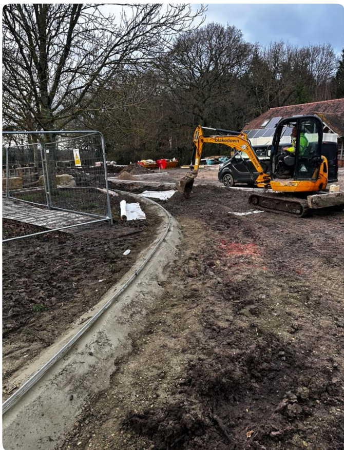
Curved edging haunched with concrete
