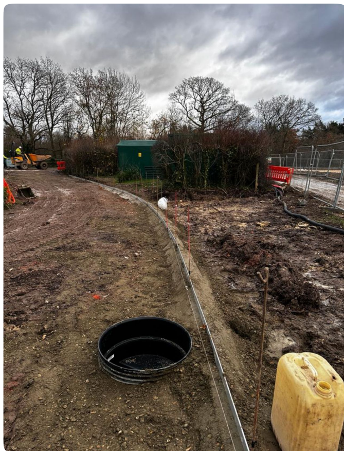
Edging follows the new path alignment
