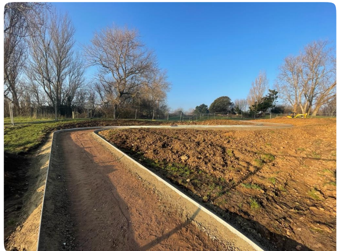
A consistent edge along the path
