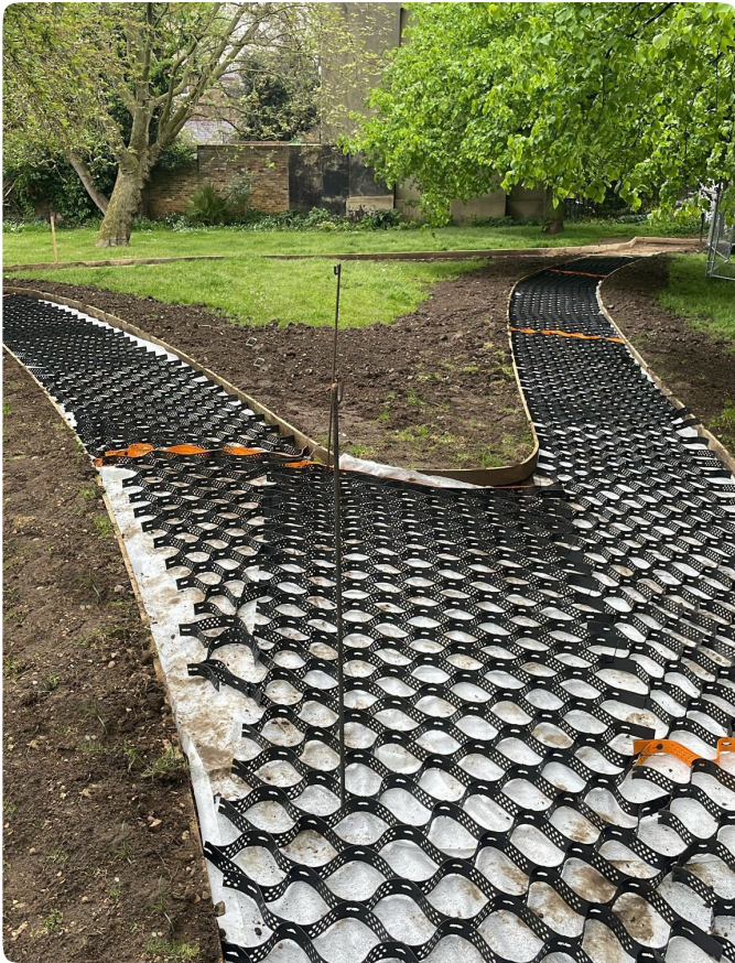
CORE TRP laid out at a path junction
