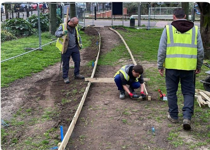
Setting out the path before CORE TRP installation
