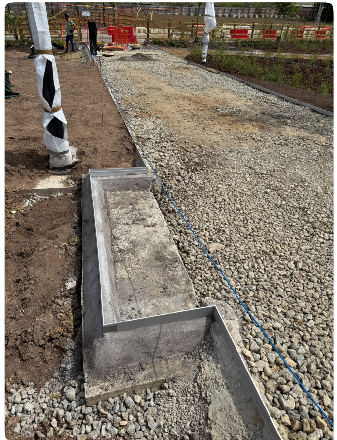
Edging haunched with concrete.
