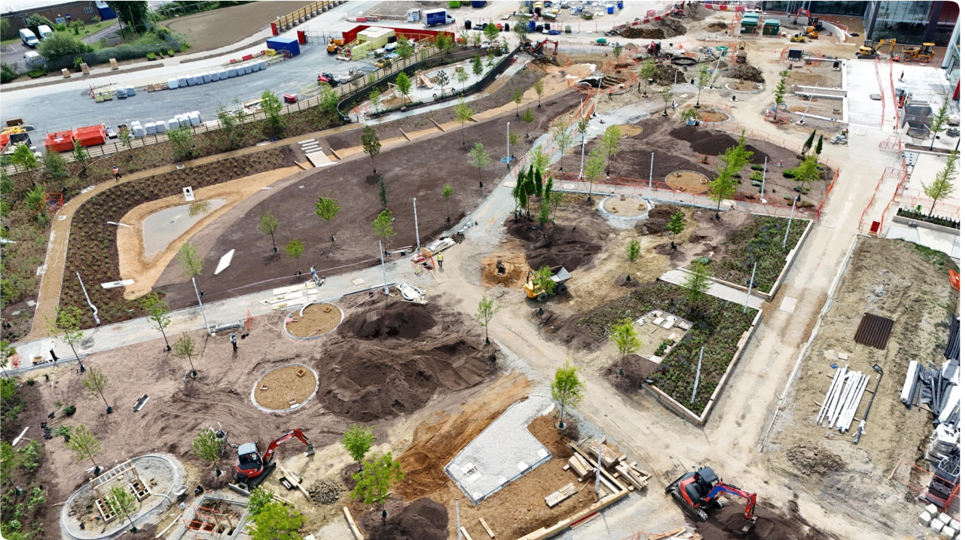
Paths and planted areas taking shape during construction.
