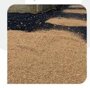
Fill the grid with your chosen aggregate using either a wheel barrow or direct from a truck.
