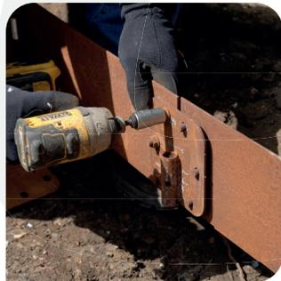
Attach the next length of edging by aligning it with the previously installed section. Use the joining plates provided to connect the two sections securely. Continue this process, attaching and adjusting additional lengths as required.
