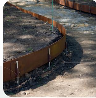
If you want to create a curve, use the ground pins to establish anchor points along the desired path. Make sure that the welded tubes are positioned on the least visible side to maintain a clean appearance.
