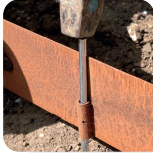
Place DATUM EDGE into the desired position. Use the ground pins provided to fix the edging into place, by inserting them through the welded tubes.
