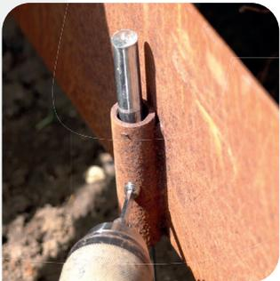
Once the edging is in place, adjust the height by sliding the edging up or down on the pins. This allows you to create your datum, ensuring the edging is level and at the correct height. Once the desired height is achieved, lock it in place using the DatumLock™ screws.
