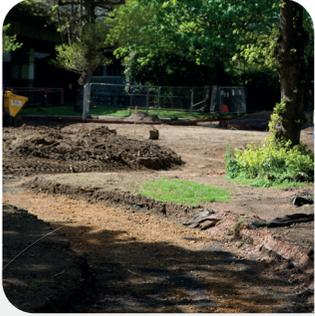
Begin by clearing the site thoroughly and preparing the sub-base as necessary to ensure a stable foundation for the edging.
