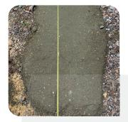
Lay a 20-30mm sharp sand/cement dry mix bedding layer onto the compacted subbase and trowel to a continuous even level. Measure down from your line at intervals to check your firmed bedding layer is at the correct level for your edging height.
