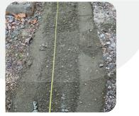
Add a further 10mm sharp sand/cement dry mix bedding layer for the CORE PRO EDGE to be laid upon.
