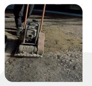
Lay and thoroughly compact your sub-base material (e.g type one limestone) to the engineers specification. Sub-base material should extend around 100/150mm beyond the proposed line of the edging.
