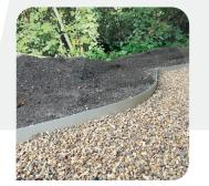
If laying against soil for turfing or planting, create a shallow haunch towards the back of the edging onto and over the foot covering the fixing pins and smooth with a trowel.
