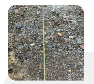
Set up a string line at the desired finish height for the top of the edging.
