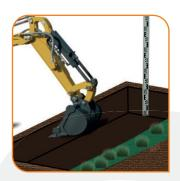
Excavate the area for your subbase to be installed. Ensure to allow an additional 10mm for the sharp sand bedding layer, 20mm for depth of grid and 10-15mm for a dressing of aggregate.
