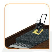
Install membrane and geogrid if required and then the subbase material. Ensure subbase is well compacted using either a pedestrian roller or vibrating road plate.
