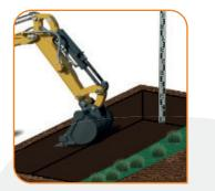
Excavate the area for your subbase to be installed. Ensure to allow for 10m sand bedding layer, depth of grid and the 10-15mm dressing of aggregate when calculating depth from surrounding surfaces.
