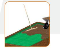
Fill the grids with soil and damp down with water to allow soil to settle into the cells. Seed the area and water thoroughly. To aid grass growth, cover the seed with a top layer of fertilizer and water regularly for a period of 4 to 6 weeks.
