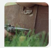
Complete the Dual Lock Mechanism® by bending back the folding tabs with your pliers.
