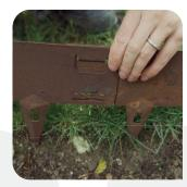
Bring your next piece and connect the two together by using the first connection at the top of each piece of edging.
