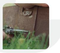
Complete the Dual Lock Mechanism® by bending back the folding tabs with your pliers.
