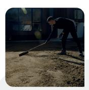
Excavate the area for your subbase to be installed. Ensure to allow for 10m sand bedding layer, depth of grid and the 10-15mm dressing of aggregate when calculating depth from surrounding surfaces. Once done, compact and smooth out the area.
