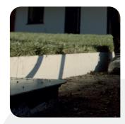
Install membrane and geogrid if required and then install a suitable edging around all open sides. This could be tanalised wood edging, block paviours, granite setts or our very own edging variations (CORE PRO EDGE shown here). Set edging 15-20mm below grid level to prevent gravel spilling out to surrounding areas.
