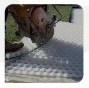
Install your CORE DRIVE sheets starting from one corner and working your way out with the membrane facing down. This particular grid has a clipping mechanism to join each sheet. Cut to shape using a petrol disc cutter or grinder. Please ensure to wear the necessary PPE for the equipment being used.
