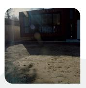
Excavate the area for your subbase to be installed. Ensure to allow for 10m sand bedding layer, depth of grid and the 10-15mm dressing of aggregate when calculating depth from surrounding surfaces.
