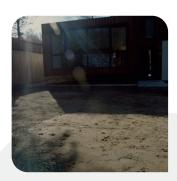
Excavate the area for your subbase to be installed. Ensure to allow for 10mm sand bedding layer, depth of grid and a 10-15mm dressing of aggregate when calculating depth from surrounding surfaces.
