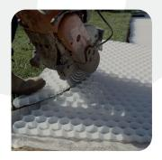
Install your CORE DRIVE sheets starting from one corner and working your way out with the membrane facing down. Cut to shape using a petrol disc cutter or grinder. Please ensure to wear the necessary PPE for the equipment being used.
