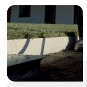
Install membrane and geogrid if required and then install a suitable edging around all open sides. This could be tanalised wood edging, block paviours, granite setts or our very own edging variations (CORE PRO EDGE shown here). Ensure to set your edging height 15-20mm higher than the grid level to prevent the dressing layer spilling out onto surrounding areas.
