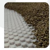
Fill the grid with your chosen aggregate using either a wheel barrow or direct from a truck. Ensure the truck does not drive onto the unfilled grid. CORE DRIVE is designed to be covered by a 10-15mm dressing layer of aggregate - making the grid virtually invisible.
