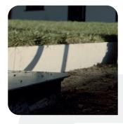
This could be tanalised wood edging, block paviours, granite setts or our very own edging variations (CORE PRO EDGE shown here). Ensure to set your edging height 15-20mm higher than the grid level to prevent the dressing layer spilling out onto surrounding areas.
