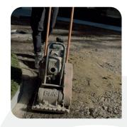
Repair the surface if there are any dips or pot holes with a suitable subbase material and recompact the entire area with a roller or vibrating road plate. If installing over tarmac or concrete, you may want to drill drainage holes in the surface to allow water infiltration.
