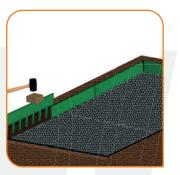
Install a suitable edging around all open sides. This could be a tanalised wooden edging, block paviours, granite setts, concrete path edgings or our very own flexible steel edging - CORE EDGE.
