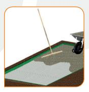
Fill the grid with your chosen aggregate either using a wheelbarrow or direct from a truck. Ensure the truck does not drive onto the grid. CORE PATH PRO is designed to be covered by a 10-15mm dressing layer of aggregate, making the grid virtually invisible. We recommend any angular aggregate up to 14mm in size.
