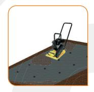
Repair the surface if there are any dips or pot holes with a suitable subbase material and recompact the entire area with a roller or vibrating road plate. If installing over tarmac or concrete, you may want to drill drainage holes in the surface to allow water infiltration.
