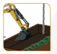
Excavate the area for your subbase to be installed. Ensure to allow for 10m sand bedding layer, depth of grid and the 10-15mm dressing of aggregate when calculating depth from surrounding surfaces.
