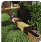
Using your block of wood and lump hammer, tap the edging into the ground to your desired height.
