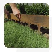
Set up a string line at the desired finish height for the top of the edging and install your first length.
