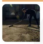
Excavate the area for your subbase to be installed. Refer to our subbase calculation guide for depth required. Ensure to allow for 10mm sand bedding layer, depth of grid and a 10-15mm dressing of aggregate when calculating depth from surrounding surfaces. Once finished, compact and smooth out the area.
