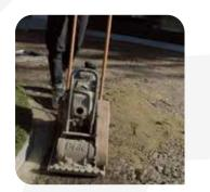
Repair the surface if there are any dips or pot holes with a suitable subbase material and recompact the entire area with a roller or vibrating road plate. If installing over tarmac or concrete, you may want to drill drainage holes in the surface to allow water infiltration.
