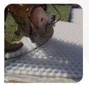
Install your CORE DRIVE sheets starting from one corner and working your way out with the membrane facing down. Cut to shape using a petrol disc cutter or grinder. Please ensure to wear the necessary PPE for the equipment being used.
