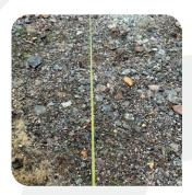
Set up a string line at the desired finish height for the top of the edging.
