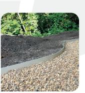
If laying against soil for turfing or planting, create a shallow haunch towards the back of the edging onto and over the foot covering the fixing pins and smooth with a trowel.
