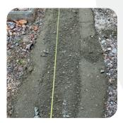
Add a further 10mm sharp sand/cement dry mix bedding layer for the CORE PRO EDGE to be laid upon.
