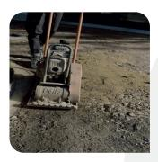
Lay and thoroughly compact your sub-base material (e.g type one limestone) to the engineers specification. Sub-base material should extend around 100/150mm beyond the proposed line of the edging.
