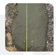
Lay a 20-30mm sharp sand/cement dry mix bedding layer onto the compacted subbase and trowel to a continuous even level. Measure down from your line at intervals to check your firmed bedding layer is at the correct level for your edging height.
