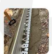
Place the edging onto the bedding layer, tap to level of the line and fix in place using the galvanised fixings through the preformed holes in the foot of the edging. Hammer fixings down securely.
