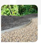
If laying against soil for turfing or planting, create a shallow haunch towards the back of the edging onto and over the foot covering the fixing pins and smooth with a trowel.
