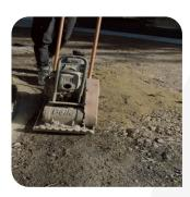
Lay and thoroughly compact your sub-base material (e.g type one limestone) to the engineers specification. Sub-base material should extend around 100/150mm beyond the proposed line of the edging.
