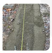
Add a further 10mm sharp sand/cement dry mix bedding layer for the CORE PRO EDGE to be laid upon.
