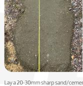
Lay a 20-30mm sharp sand/cement dry mix bedding layer onto the compacted subbase and trowel to a continuous even level. Measure down from your line at intervals to check your firmed bedding layer is at the correct level for your edging height.
