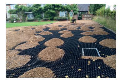
PRACTICAL | REMOVED EXISTING TARMAC, REPAIRED SOLUTION **SUBBASE, LAID CORE DRIVE 60-40 HDR**
